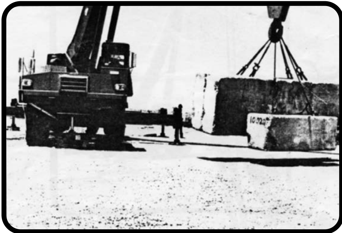
In Action. The T7580 10x4 Bucyrus-Erie 90XC combination lifts 89,425 lbs. at a 25' load radius.
