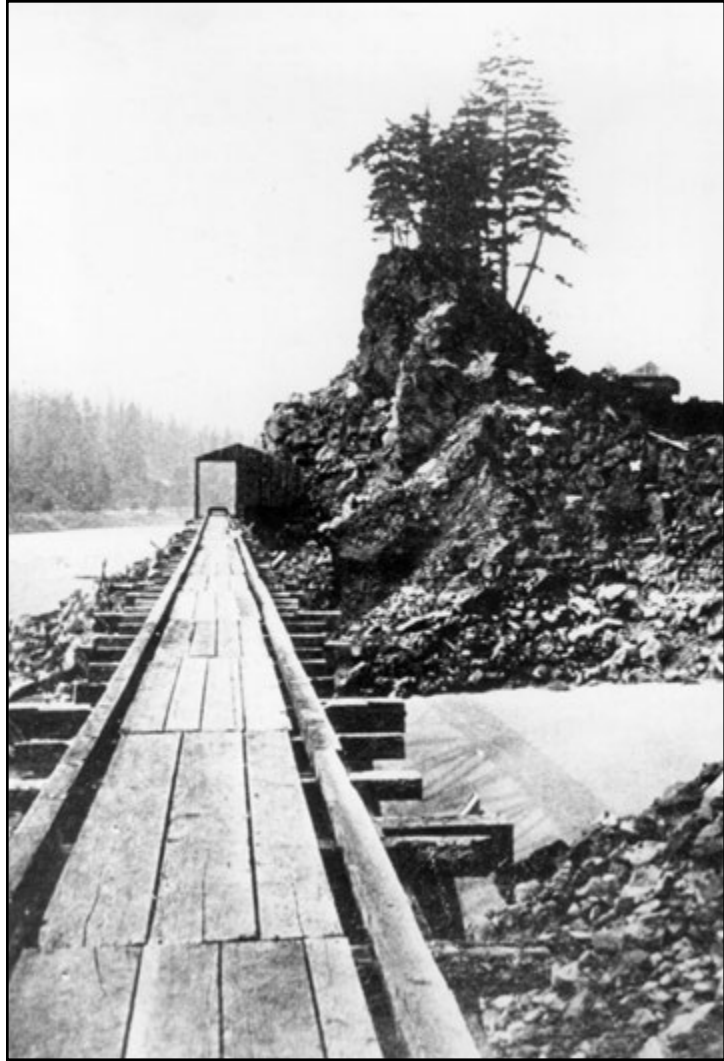
The old portage railroad, operated originally by mules or horses pulling flat-bed cars around the Cascades on a semi-circular course of six miles. Rawhide was used at first to cover the wooden rails, but wolves would chew it off. Strap iron was then used until iron T rails were laid. Fort Rains is on the hill at right center. Photo taken prior to 1876.
