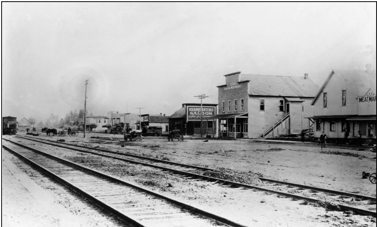
Front Avenue of Stevenson, south of the S.P.&S. railroad tracks. First building on right is the City Meat Market. Next is the C. S. Doumitt General Store. Next is the Headquarters Saloon, owned by Lew Iman. The sign says: "For Miners, Loggers and Railroaders. Our motto: Every Man's Credit Good." The last building was the Hotel Stevenson, owned by Russell and Flora Swain. (HOW ABOUT JEFFERSON NIX? ←
