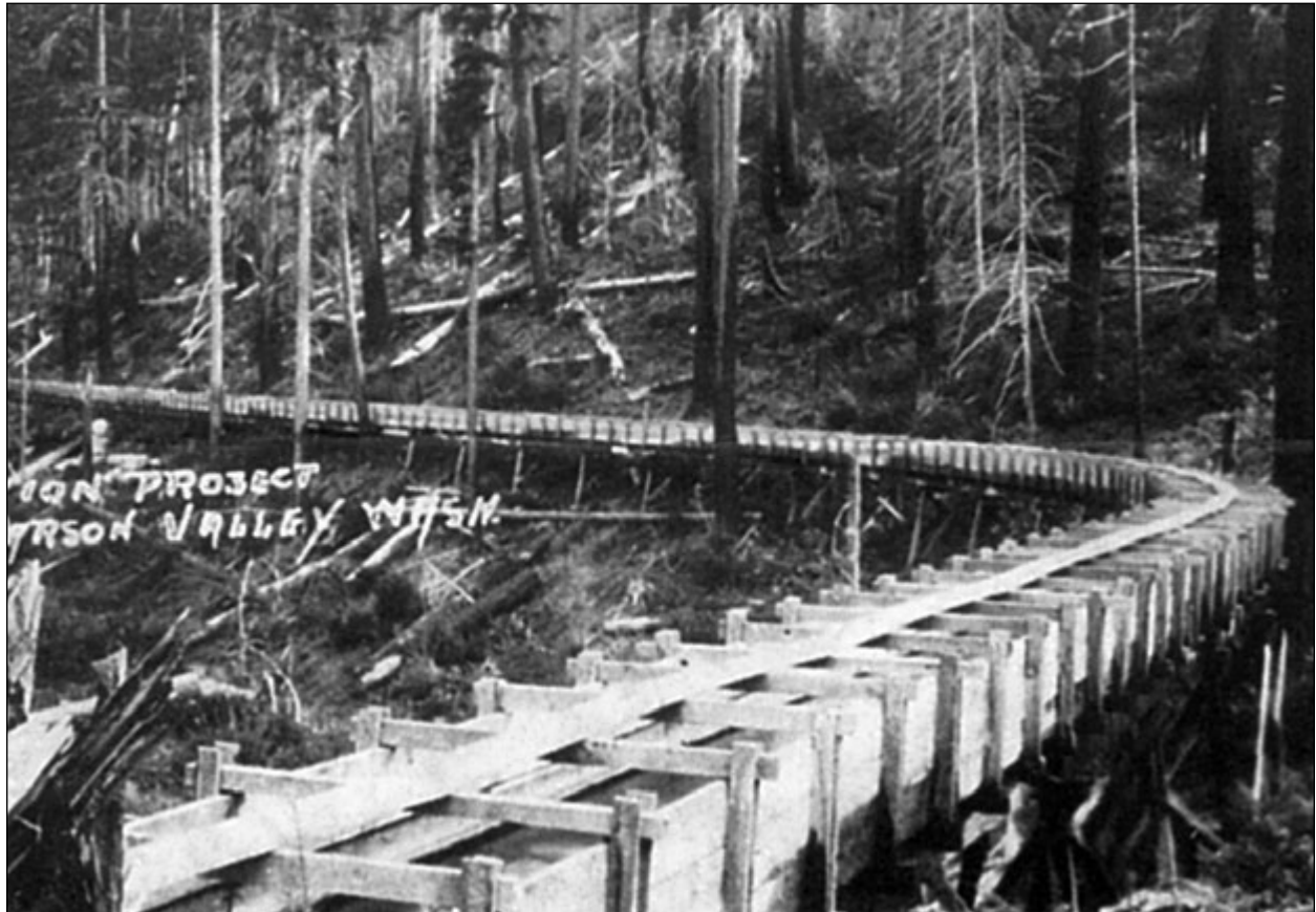
Irrigation flume wends way from Panther Creek toward yet-to-be-built High Bridge over Wind River.
