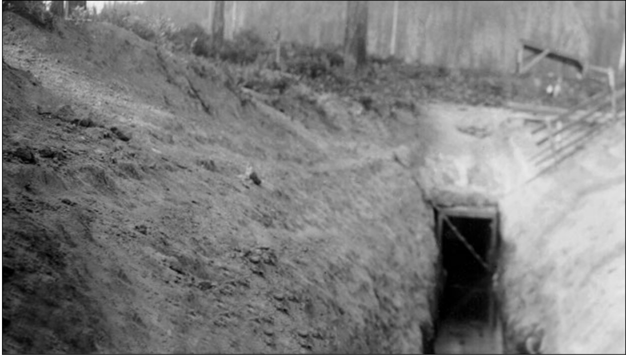
Hand-bored tunnel permits flow of water into irrigation flume.
