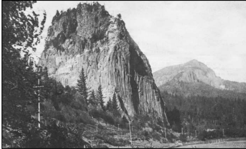
Photograph made in 1920 several years following the completion of the trail to the summit. Rock fallings are visible which resulted from the construction of steps and inclined on the trail. Today, these tailings are not as apparent since vegetation, moss, and lichens have established themselves over and on the rocks. Photograph courtesy of the Oregon Historical Society, File No. 262-1.
