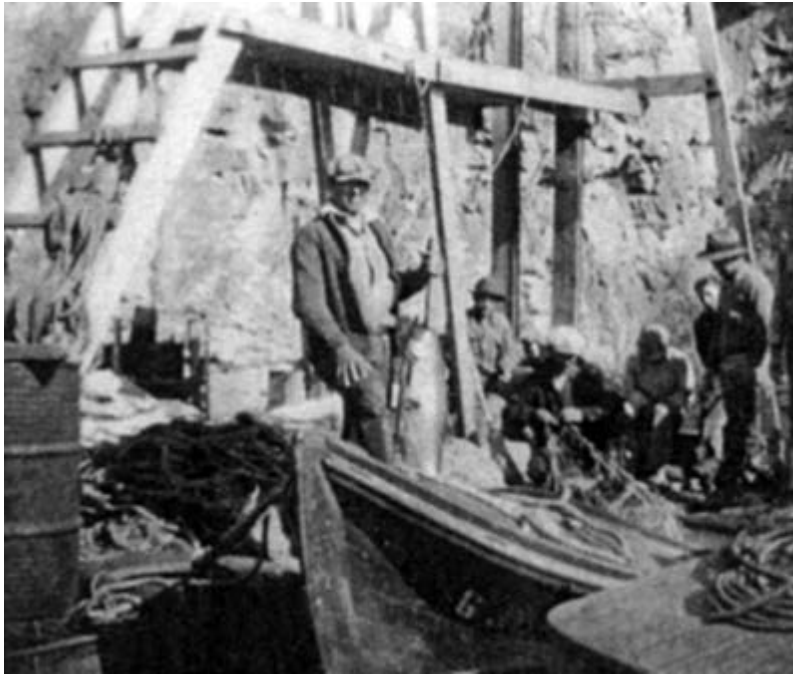
Pile driver at Lyle, Washington.
