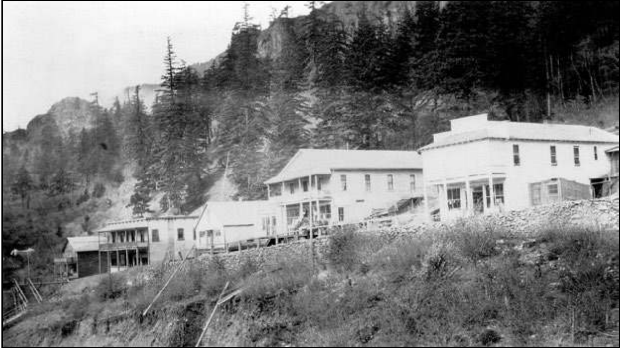
Town of Cooks, as seen from bunkers on the railroad station.
